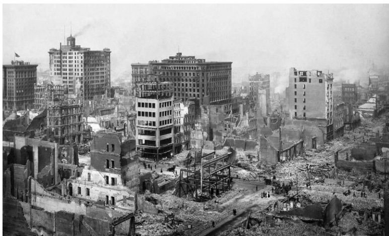
14. San Francisco earthquake damage near Post and Grant Avenues.
